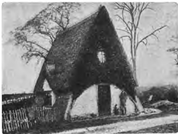
FIG. 24.—When the sapling-rafters were cut off at the ground, they ran straight to the ridge-pole. "Teapot Hall," Scriverby, England, still standing.
